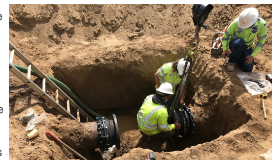
The crew working on a pipeline.
