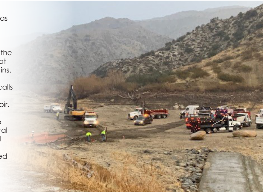
Contractors removing sediment at Littlerock Reservoir.
